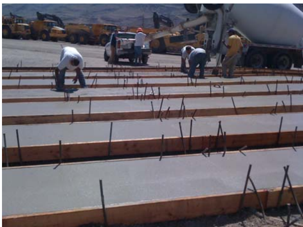
Placement of the Concrete Slabs
