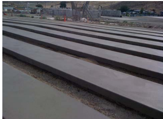
Slabs after Removal of Forms
