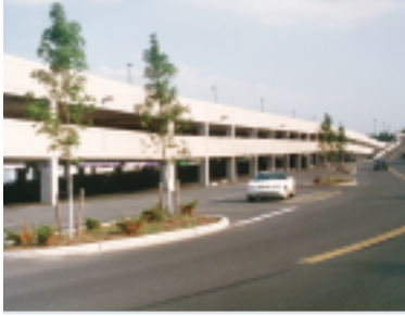
Precast Concrete Holyoke Mall Parking Garage, Holyoke, MA
